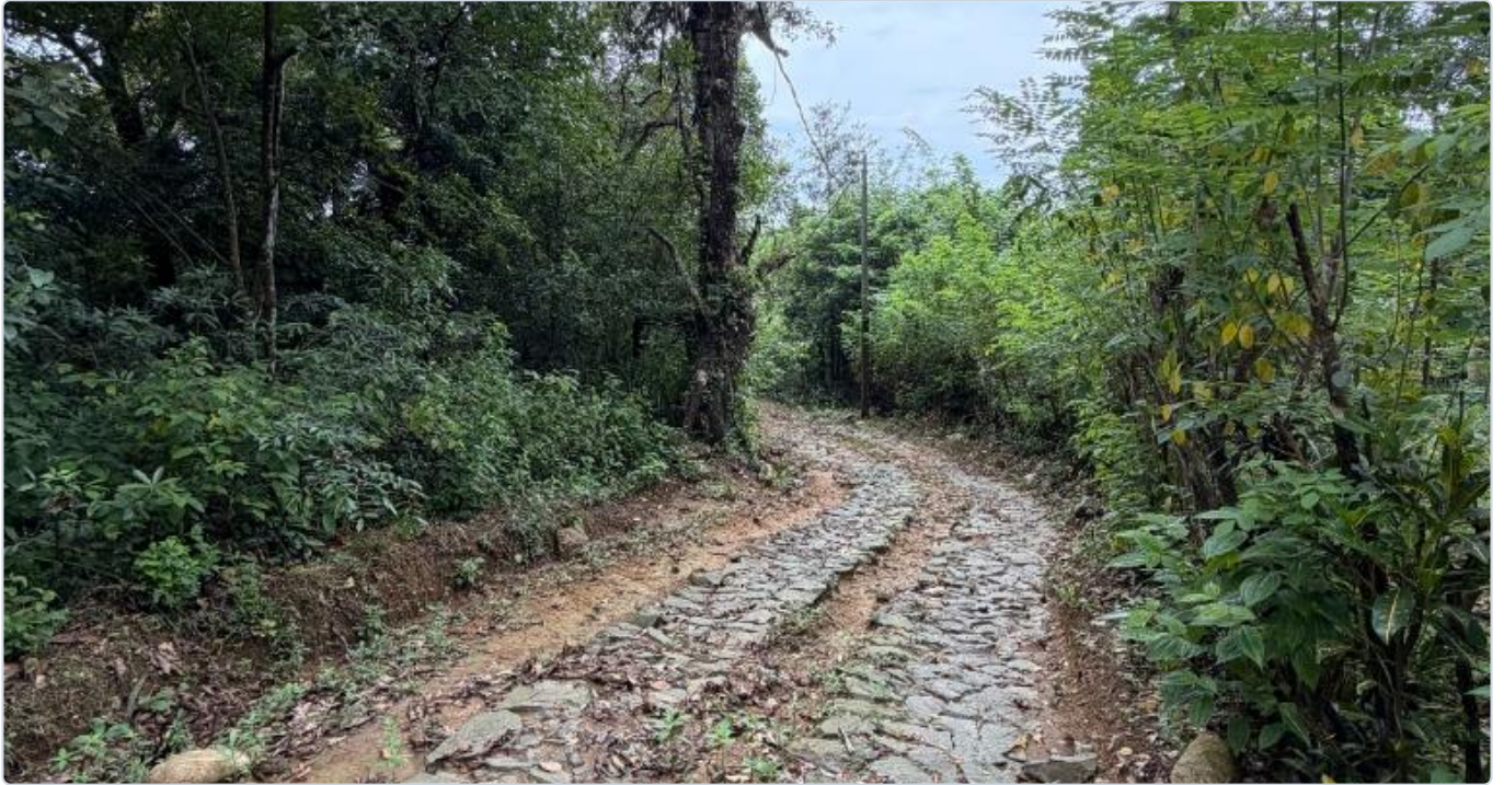
Figure 2: Custom stone-paved, all-weather interior access track entering the primary boundary line.
