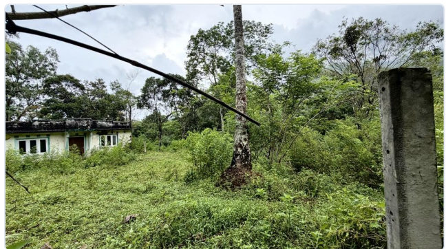
Existing concrete structures providing structural baselines for renovation or redevelopment.
